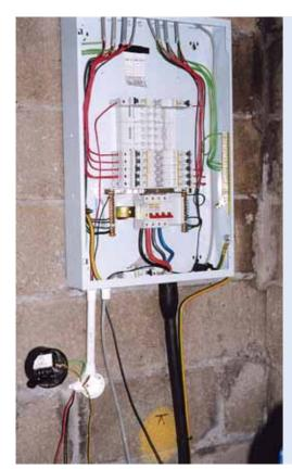
An electrician working on a new-build construction project installed the 3-phase and neutral distribution board shown in the photograph. He energised the supply to the distribution board before the circuits connected to it were complete, to provide a supply to a socket outlet.
